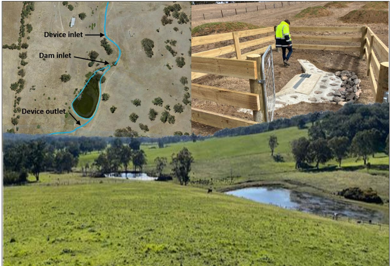
Figure 4. The preferred delivery option is a gravity low flow device (top), used in a typical a catchment setting (below).
