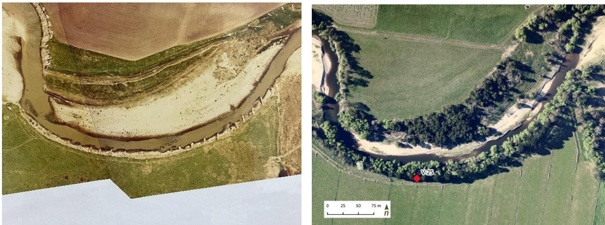
Figure 3. Early 1980's as-constructed aerial imagery of Group V groynes (left), current condition of groyne site (2018) (right)
