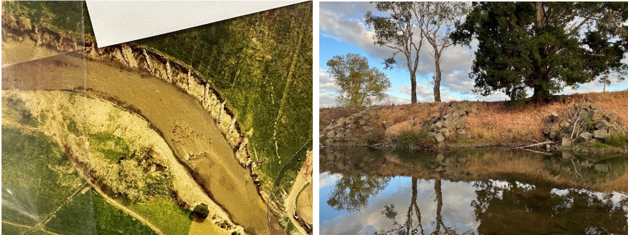
Figure 2. Early 1980's as-constructed aerial imagery of Group E groynes (left), current condition of groyne (2023) (right)
