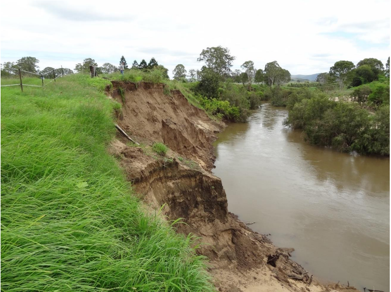
Figure 1. Site 1 prior to rehabilitation works showing extensive vertical eroding banks
