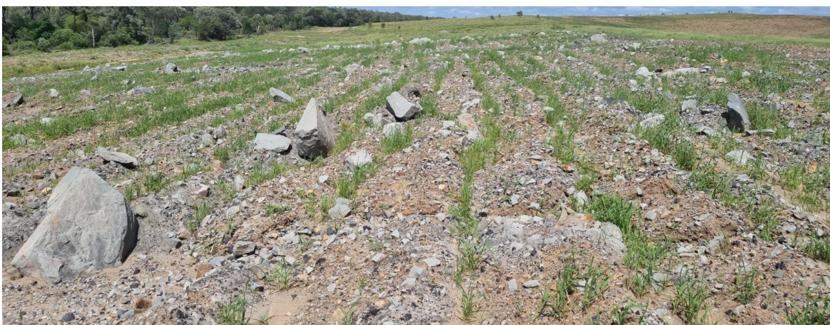
Figure 3: Spoil pile has been rock-mulched in situ (deep ripped by a dozer).
