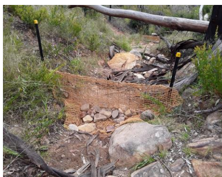
Figure 3. Example of installed channel sediment capture structures.
