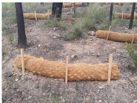
Figure 2. Example of installed coir logs.
