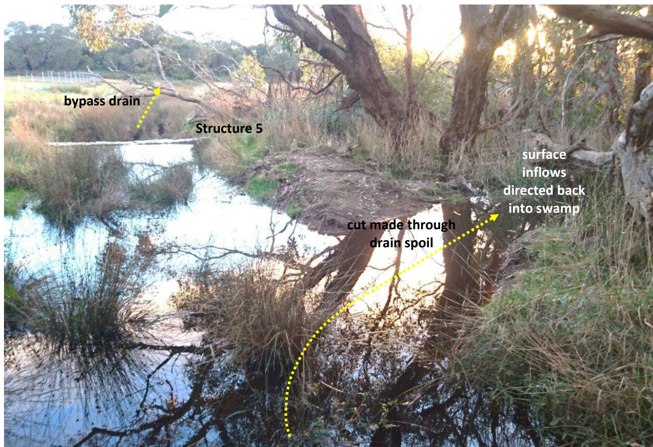
Figure 5. Surface inflows redirected back into Glenshera Swamp by Structure 5, winter 2017.
