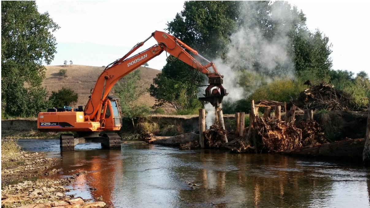
Image 1. Re-snagging and bank stabilisation on the Nariel Creek
