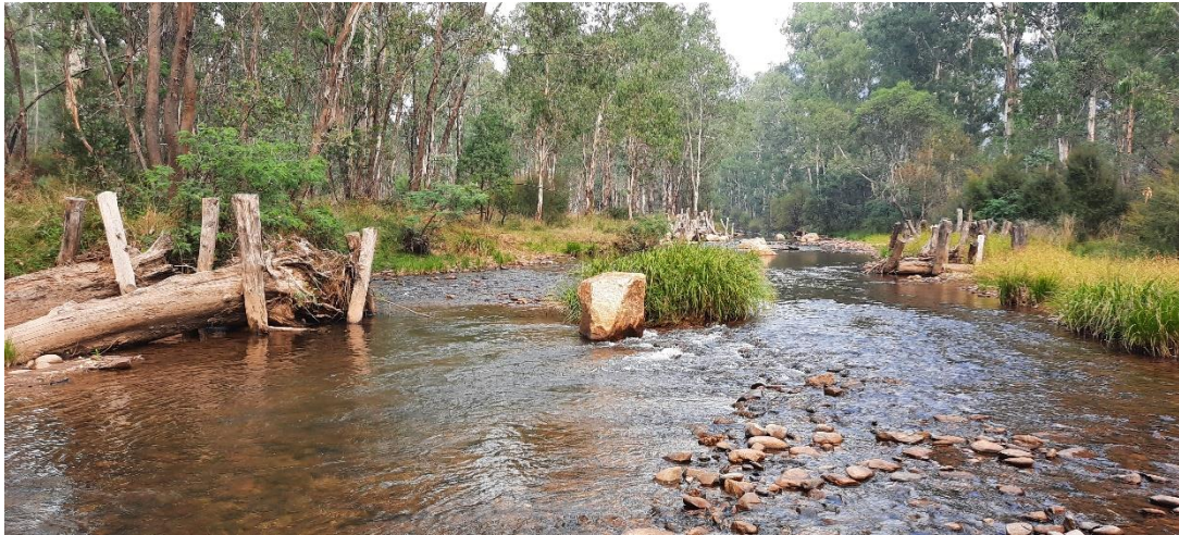
Image 2. Re-Snagging and Rock seeding on the lower Buckland River. The channels have deepened since works were completed
